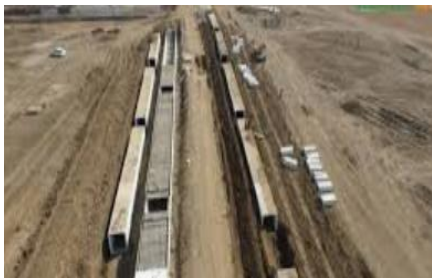
Drainage network construction
